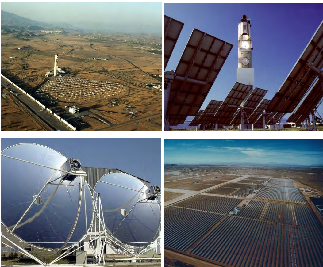
Fig. 27: Solar thermal power plant with two-dimensional tracked heliostats (top), two-dimensional tracked concentrators (bottom left) and with one-dimensional tracking by parabolic reflectors (bottom right) (Forschungs-Verbund Sonnenenergie)
