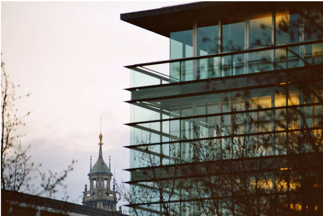
Fig. 8: Stainless steel frames in an office building façade (AEGIS Hannover, ARCASA).
