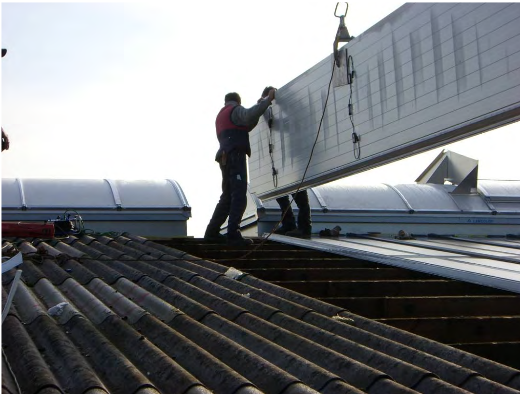
Fig. 10: Large insulated roof element (Hoesch-Contecna).
