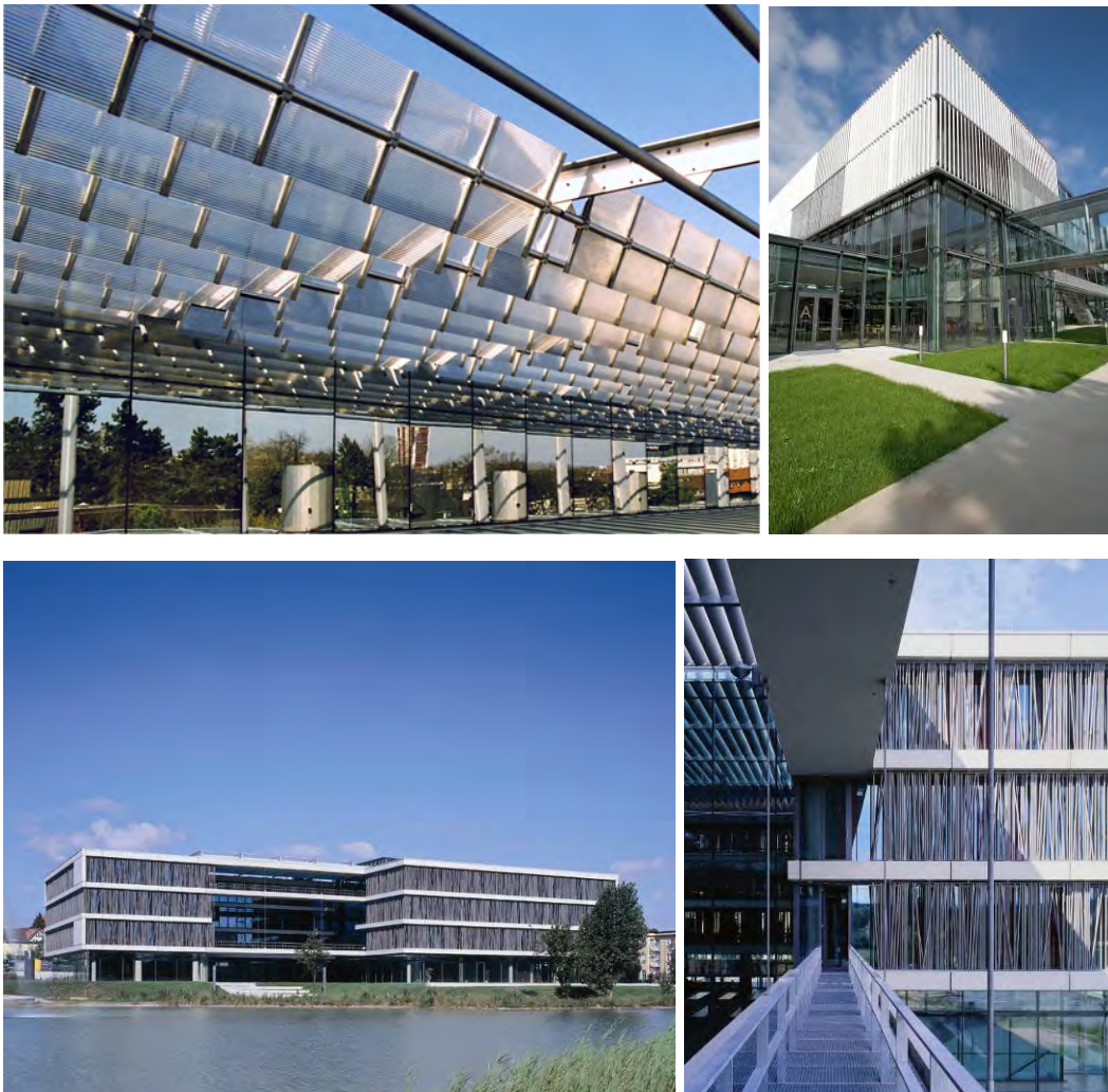
Fig. 15 Daylighting systems: prismatic louvers (top left), vertical metallic louvers (top right) and vertical daylighting devices (BKK Schweningen, bottom) (COLT BOMIN SOLAR)
