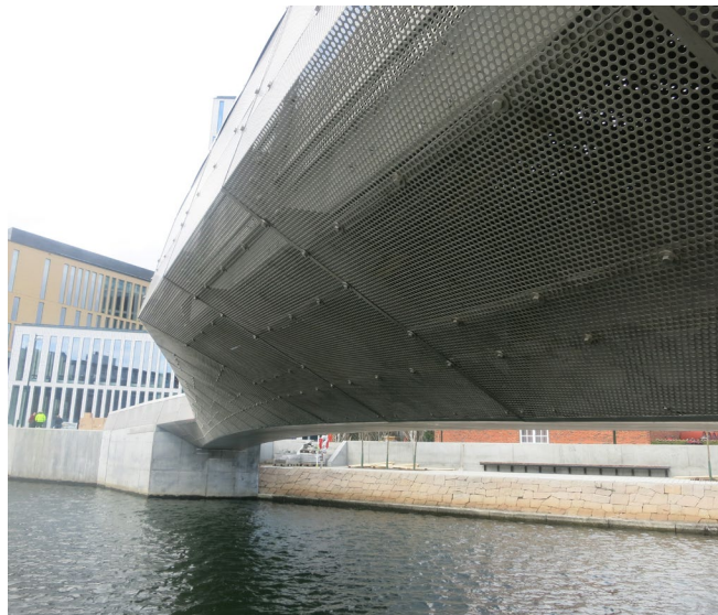
The bridge was fully pre-fabricated and transported to the site in one piece. Photos: Vistal Gdynia S.A., Gdynia, Poland
