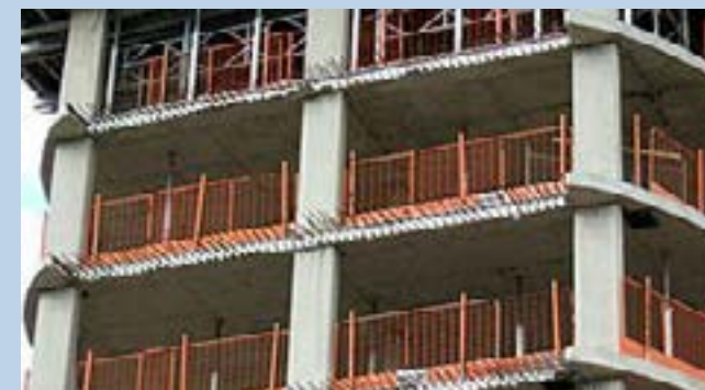
Connectors awaiting installation of the balcony
