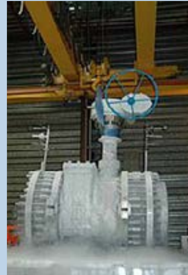
Tapped valve after testing in liquid nitrogen
