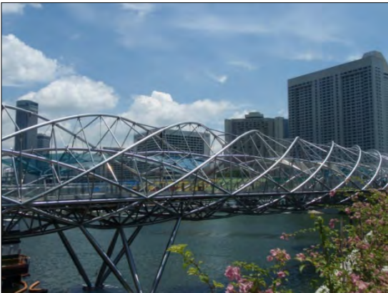
Helix Bridge, Singapore, 2011
