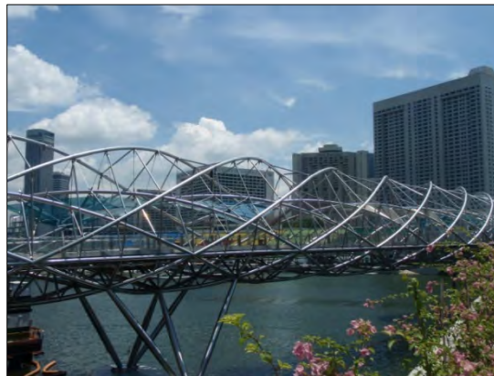
Helix Bridge, Singapur, 2011
