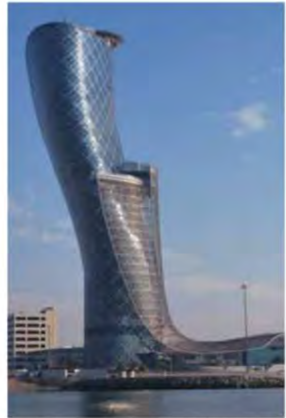
Figure 4. Woven stainless steel sweeps down from the 19 th floor of Abu Dhabi's Capital Gate Tower, reducing energy requirements. © Jeff Schofield
