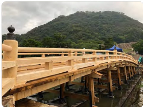
Giboshi-bashi Bridge. Picture courtesy of Tottori-city.
