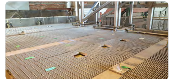
Installation of gratings. Picture courtesy of Outokumpu
