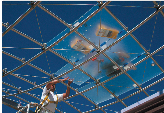
Figure 8: Placement of the glass panels (Photo: The Schubert Club)
