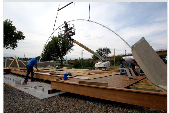
Figure 5: Installation of the first curved member (Photo: The Schubert Club)
