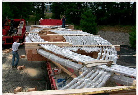
Figure 4: Curved members ready to be delivered to site (Photo: Tim Eliassen)
