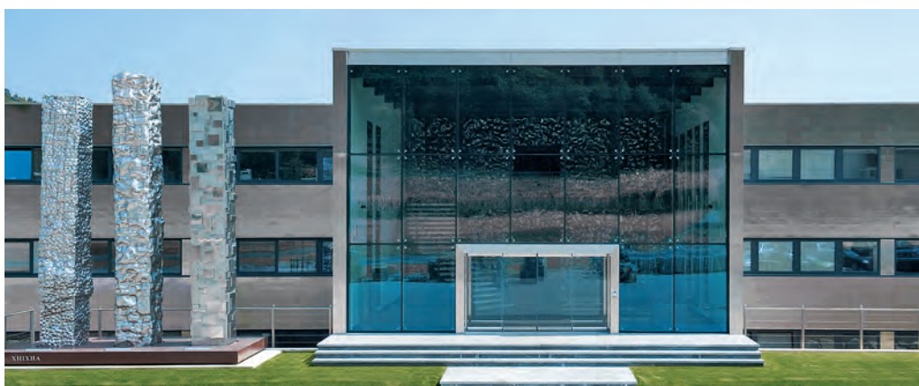
Façade of grade 1.4162 duplex stainless steel Photo: Montanstahl, Stabio (CH)
