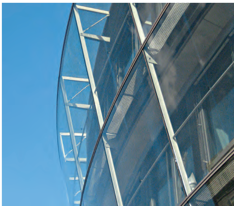
Work-hardened stainless steel grade 1.4571 of the strength class +CP350 was used in the structure of this stainless steel and glass façade.
