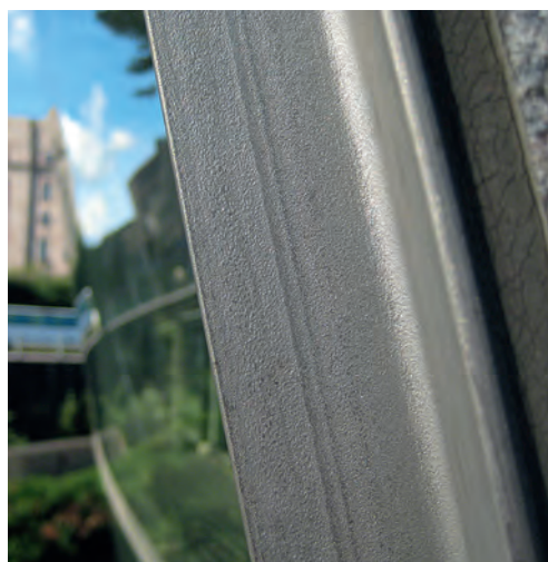
Hot rolled stainless steel with a 1D finish in an L profile on a glazed façade
