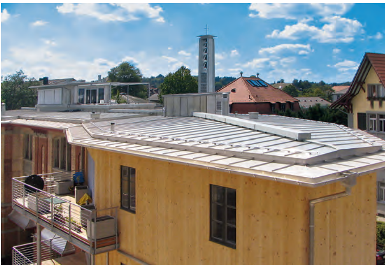
Grade 1.4510 ferritic stainless steel with an additional tin coating develops a decorative non-reflective patina over time. Photo: Blum & Rossbacher/Aperam, Luxembourg (L)
