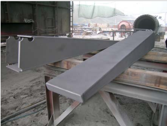
Figure 8: Final surface finish on structural members
