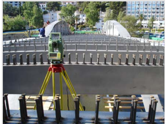
Figure 12: Shear connectors on transverse beams
