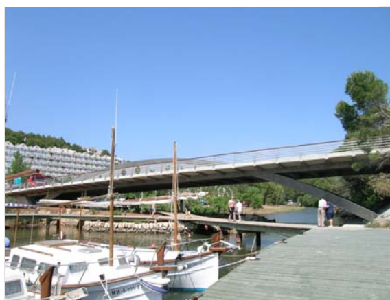
Figure 1: General view of the bridge
