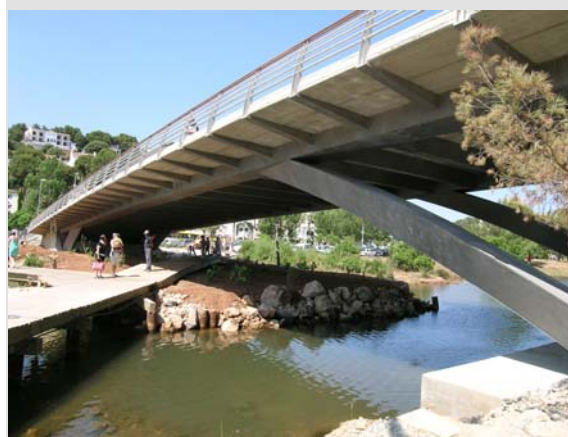
Figure 2: Arch-longitudinal beam connection
