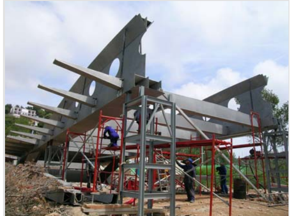
Figure 11: Temporary supports for the main structure
