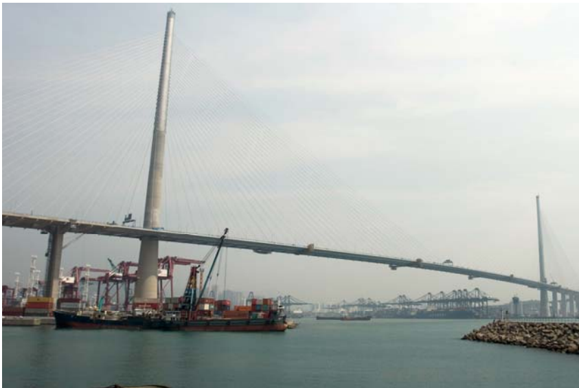
Figure 1: General view of Stonecutters Bridge
