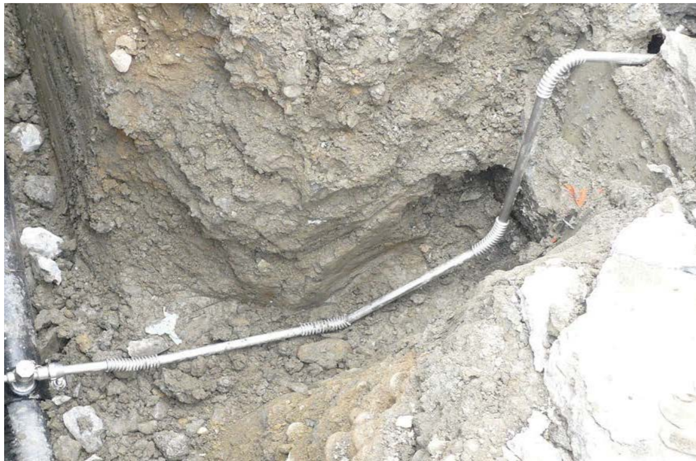
SPCT can be bent at each corrugated section. In the lay-out shown, no bends are made at the tapping valve. A 90 degree bend is easily made at the meter connection.
