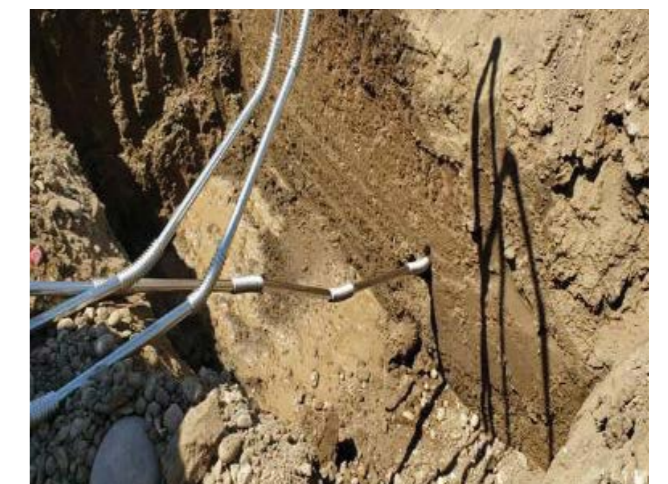
Single SPCT lengths can be orbitally welded into coil and can be installed in a trenchless way.
