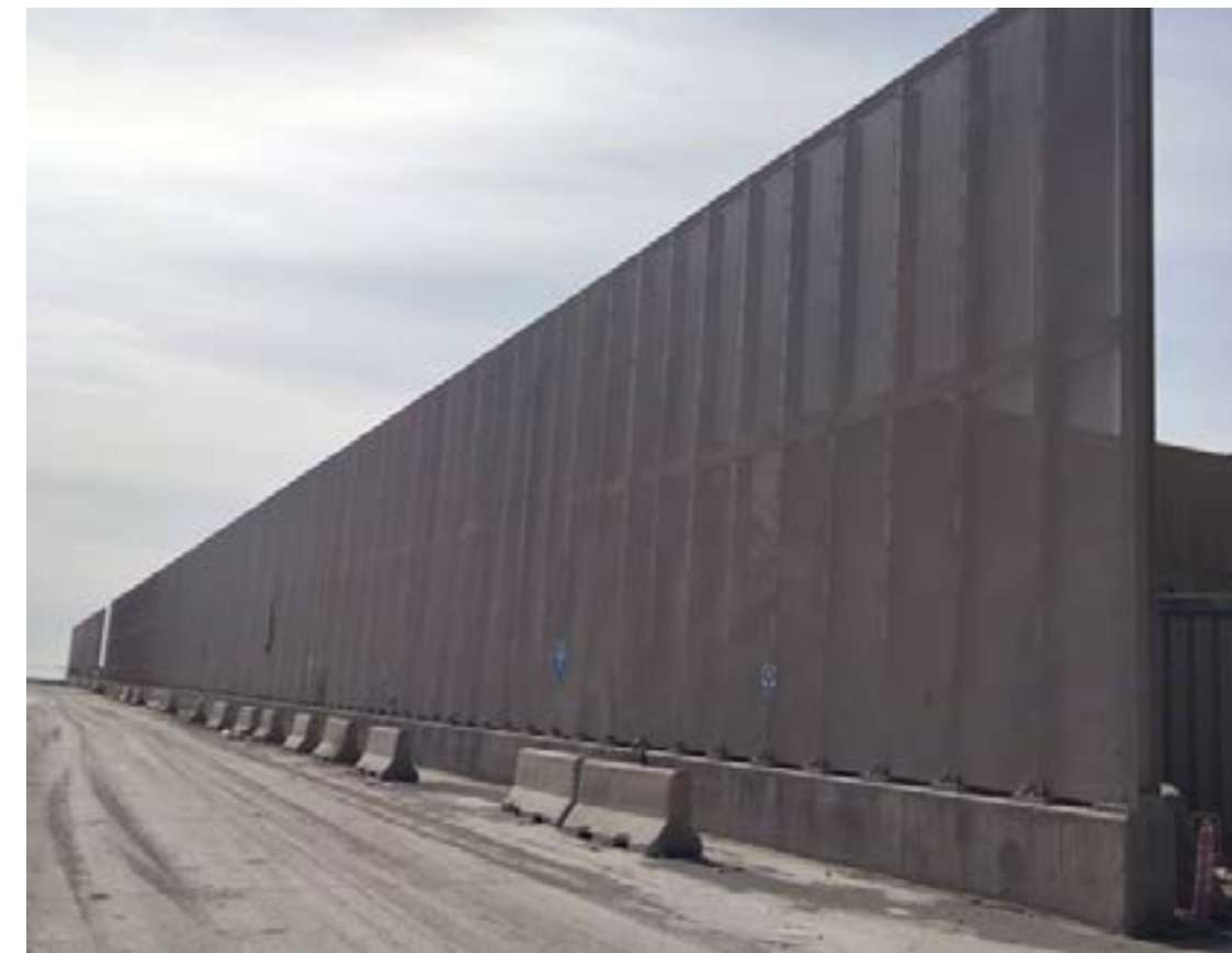
Image 3. Environmental dust retention screens.
