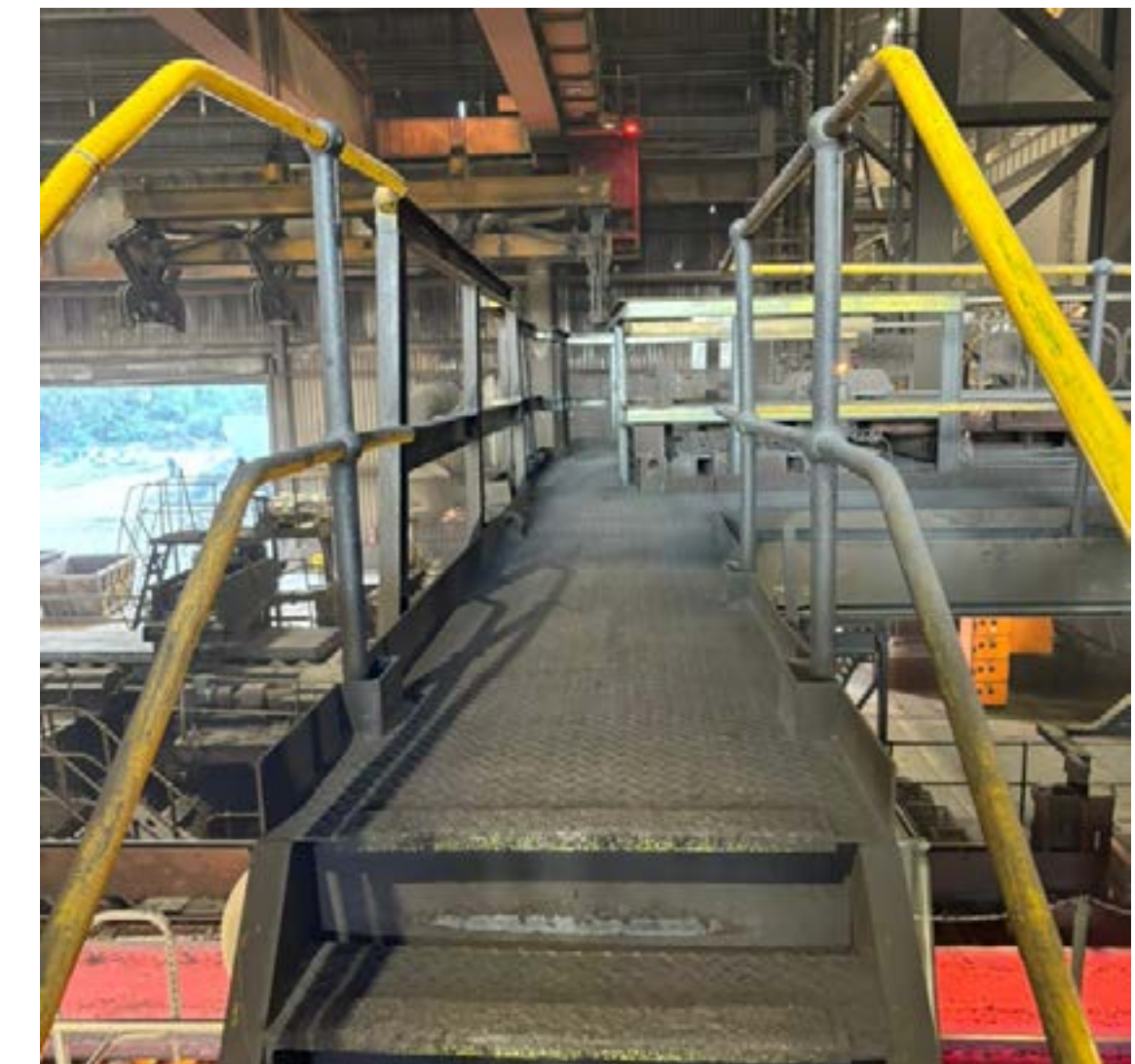
Walkway passing over the slab cutting area
