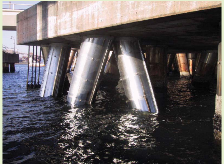
Use of grade 185N (UNS S31254) protects harbour installations
