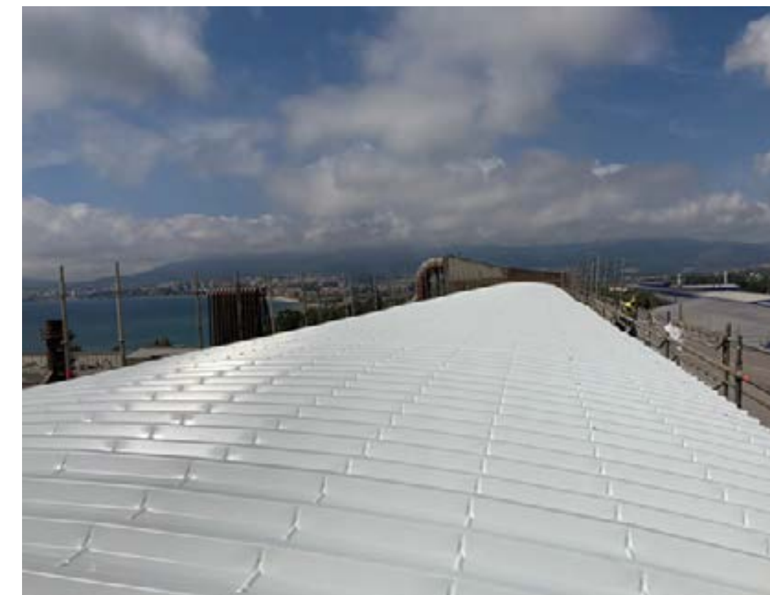
Image 4. Closing ceiling aerators in Steel Plant.
