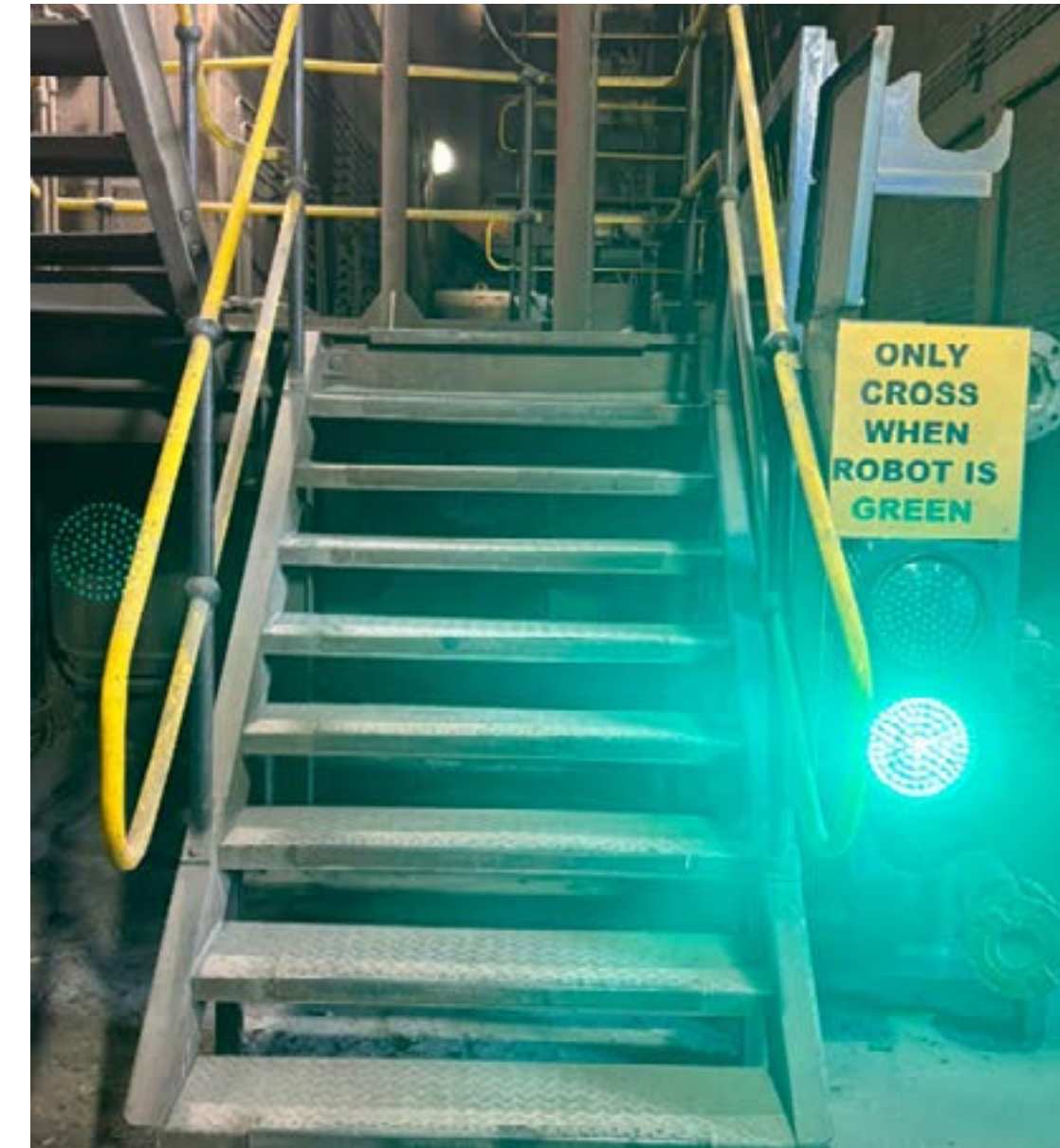
Green Robot at one of the walkway access point indicating safe passage
