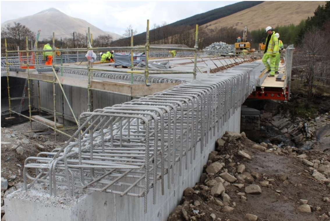
Wing walls and bridge deck under construction using stainless steel rebar
