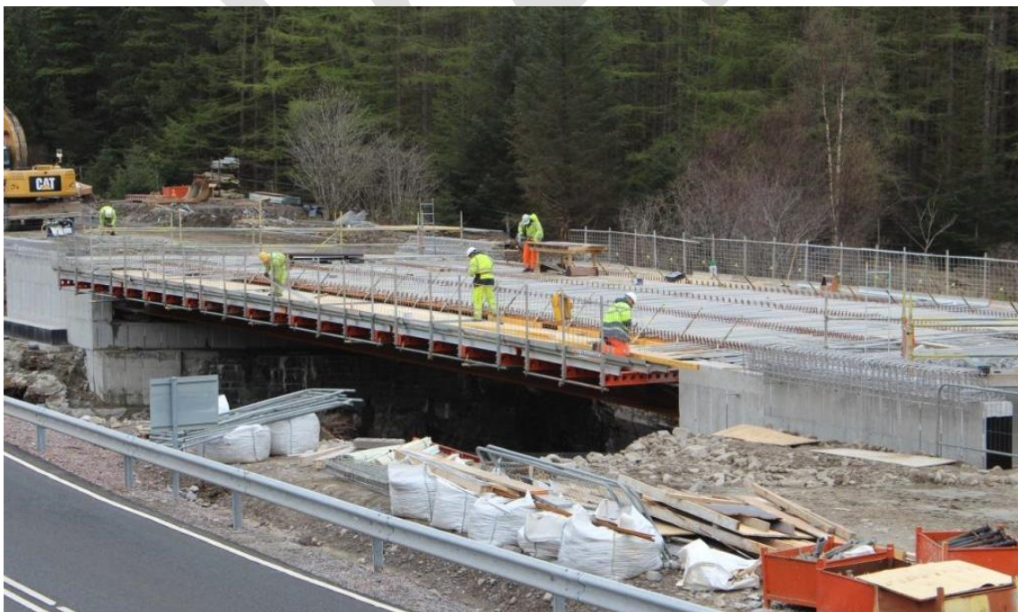
New Bridge under construction
