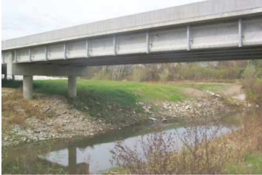
Figure 10.b. Photograph of Bridge #2.
