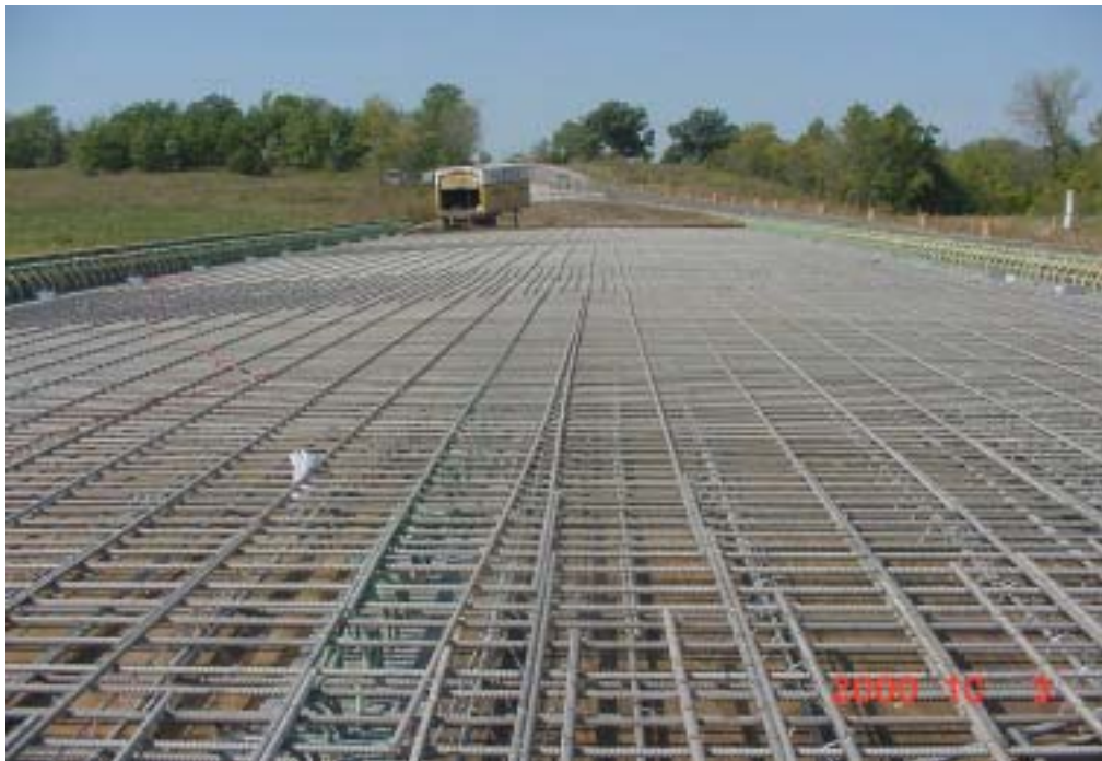
Figure 1. Stainless Steel Reinforcement of Bridge A6059
