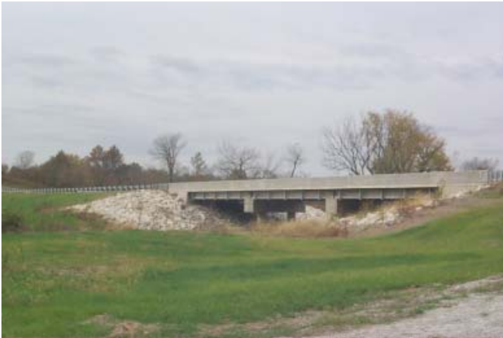
Figure 10.a. Photograph of Bridge #1.
