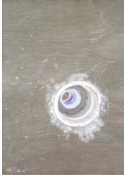
Figure 15. View of an exposed sensor housing located in bridge#1.
