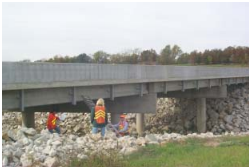
Figure 14. Ladders provided access to the sensor housings.
