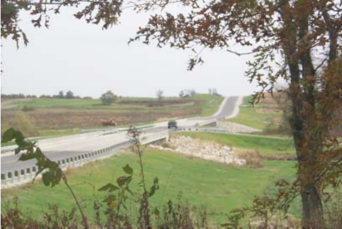
Figure 9. View of the twin State Highway 6 bridges located near Galt, Missouri.
