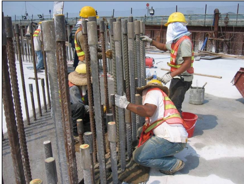
Figure 7.1 Fixing Stainless Steel reinforcement for the columns on Stonecutters Bridge
