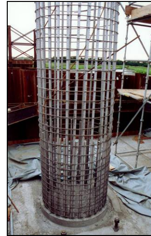
Figure 7.3 Broadmeadow Bridge and detail of stainless steel reinforcement cage for columns
