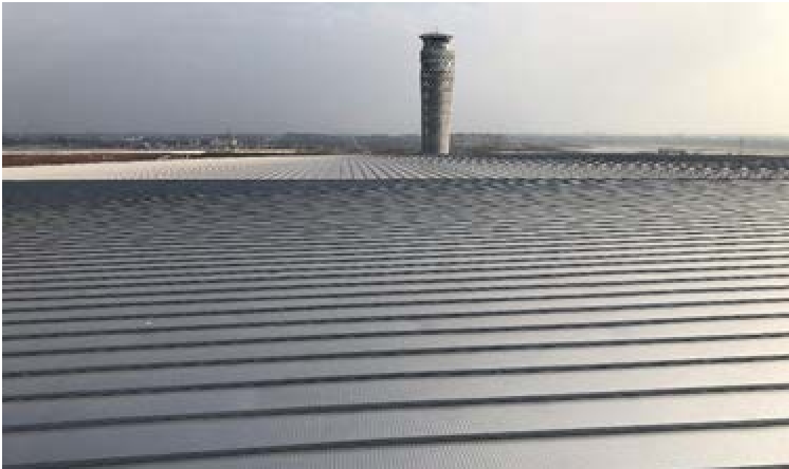
Qingdao Jiaodong International Airport welded stainless steel roof (stainless steel thickness 0.5mm) Picture courtesy of the Stainless Steel Council of China Iron and Steel Association
