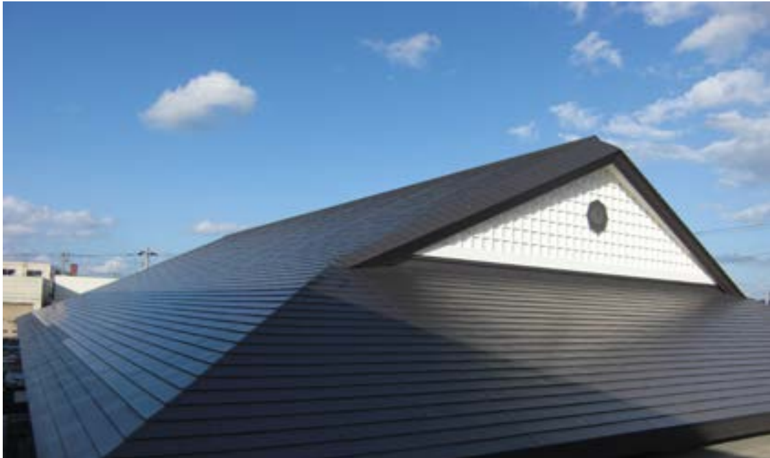
"Perfect Roof" of High-purity Ferritic Stainless Steel (SUS443J1) Picture courtesy of the Japan Stainless Steel Association
