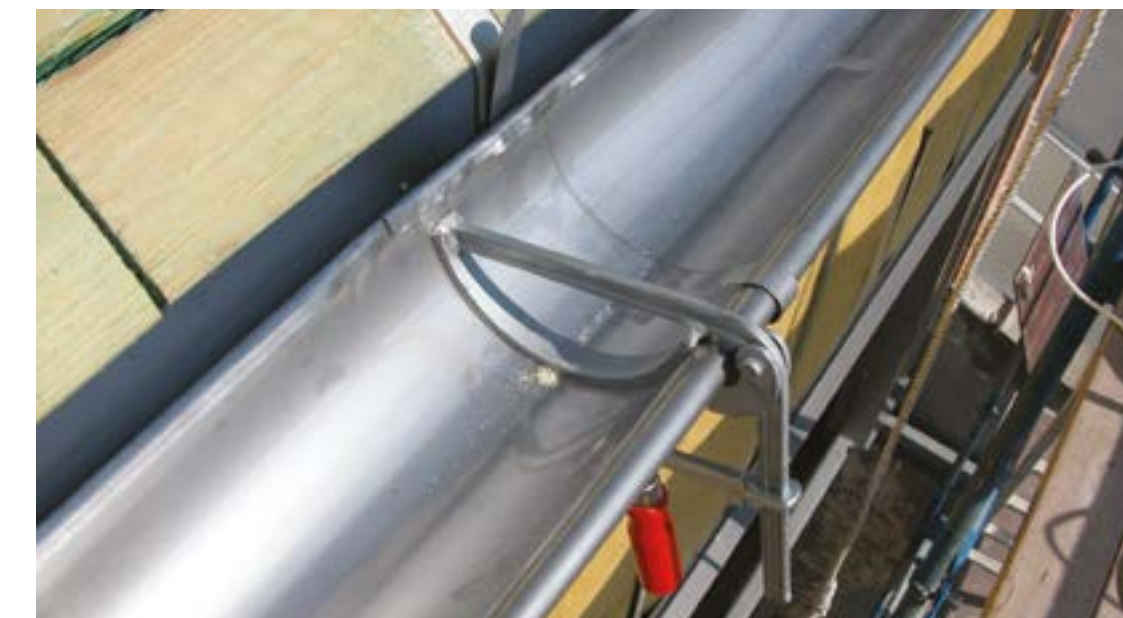
Bonding of guttering, tin-coated 430Ti. Picture courtesy of Willem de Roover, Ghent, Belgium;
