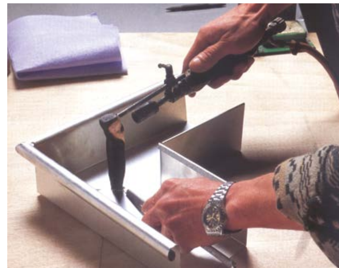
Soldering a gutter, tin-coated grade 430Ti. Picture courtesy of Brandt Edeltahldach GmbH, Cologne, Germany
