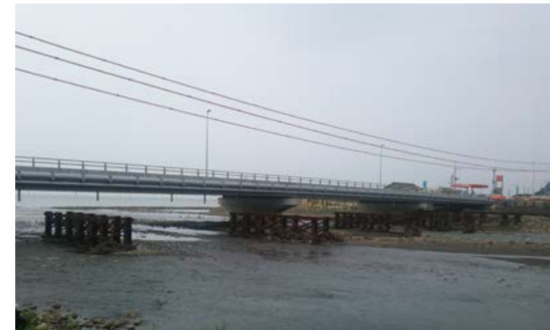
Nou Bridge - Grade SUS410 rebar Picture courtesy of the Japan Stainless Steel Association
